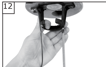
12 Loosen one and remove one preassembled screws from mounting bracket. Save screw for later use.
